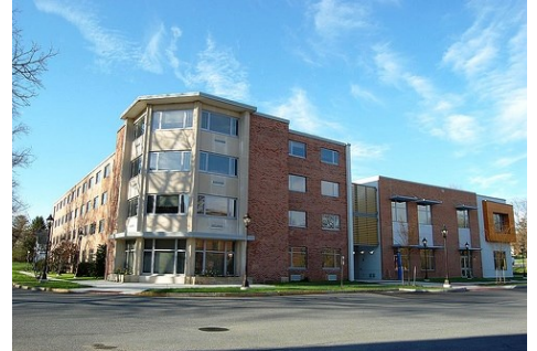
Millersville University, Stayer Hall Education Building
