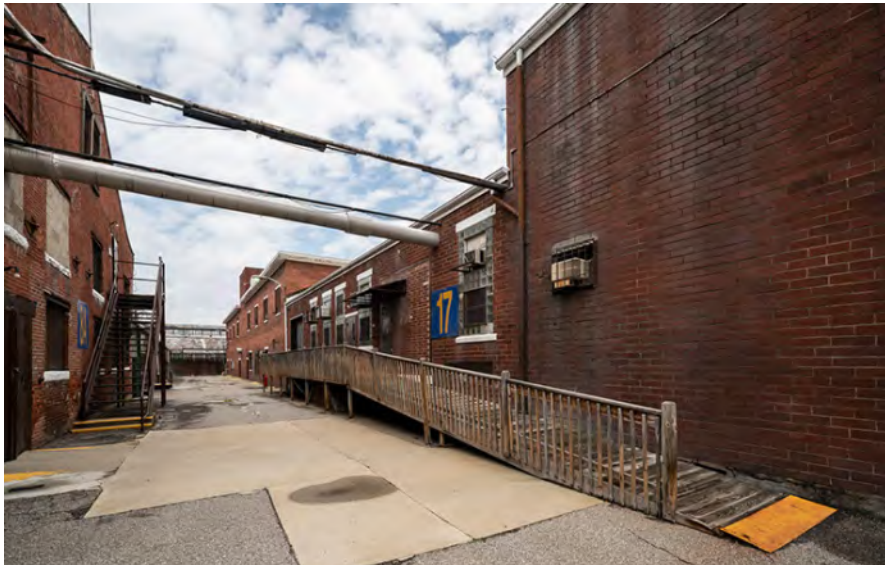
Photo 61. Maintenance Building, west facade, looking northeast.
