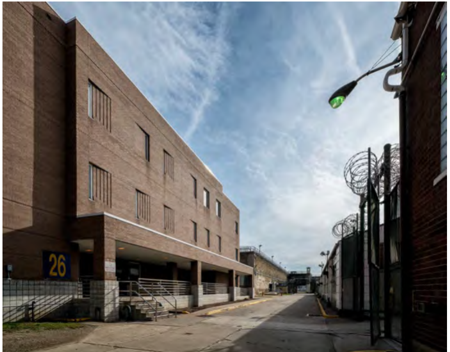
Photo 75. Health Services Building, west facade, looking southeast.
