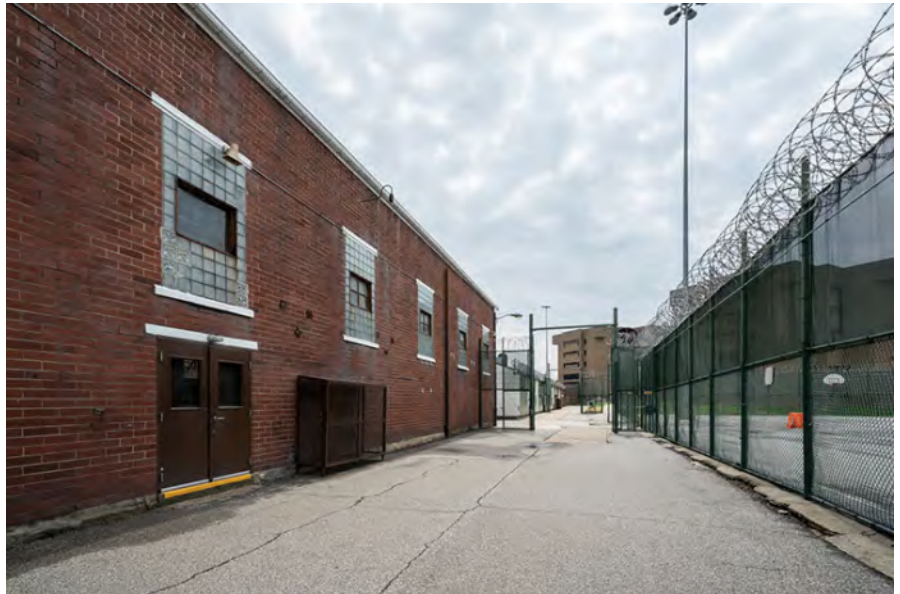
Photo 57. Gymnasium, west facade, looking southeast.
