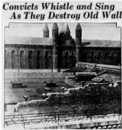
Figure 93. Newspaper headline and photograph showing the inmates deconstructing the north wall to make room for the new hospital. The area was enclosed by a new concrete rampart (The Pittsburgh Press, 4/5/1932).
