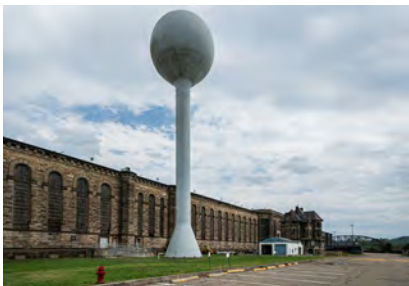
Photo 103. Water tower, looking southeast.
