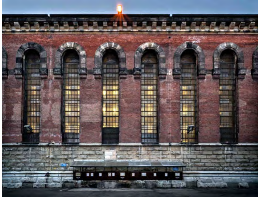
Photo 14. Main Penitentiary Building, North Wing, east facade of Housing Unit E, looking west, showing the battered stone base of the wall with arched windows and brick walls above topped by a cornice of stone modillions. Only the east facade is finished in brick; the others are clad in stone.
