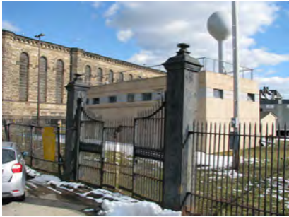
Photo 91. Cast and wrought iron gate, north side of Historic Front Yard, looking southeast (Jeff Slack).
