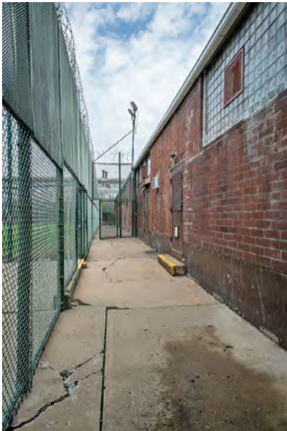
Photo 43. Services Building, west facade, looking north.
