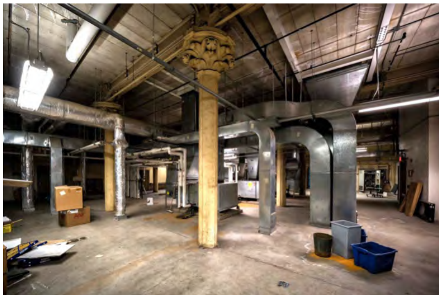
Photo 27. Main Penitentiary Building interior, fourth floor of Rotunda, looking northwest, showing the mechanical space with its floor slab that was inserted into the building in 1959 and the original cast iron columns with their decorative capitals. Similar capitals remain above the dropped ceiling on the first floor.
