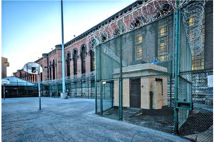
Photo 70. Inside Pump House (right), looking southwest.
