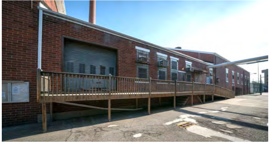
Photo 60. Maintenance Building, west facade, looking southeast, with the Gymnasium shown at the far right.
