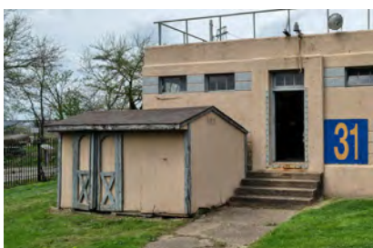
Photo 96. Shed outside Sewage Pump House, looking northwest.
