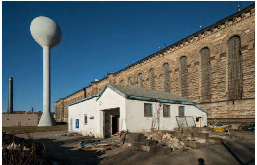
Photo 72. Storage Building, looking northeast, showing the former garage of the Warden's Residence with the North Wing of the Main Penitentiary Building and water tower in the rear.
