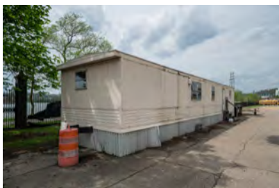
Photo 94. Modular Building (37), looking northwest.
