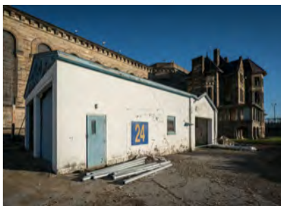
Photo 73. Storage Building, looking southeast, showing the Warden's Residence in the rear.
