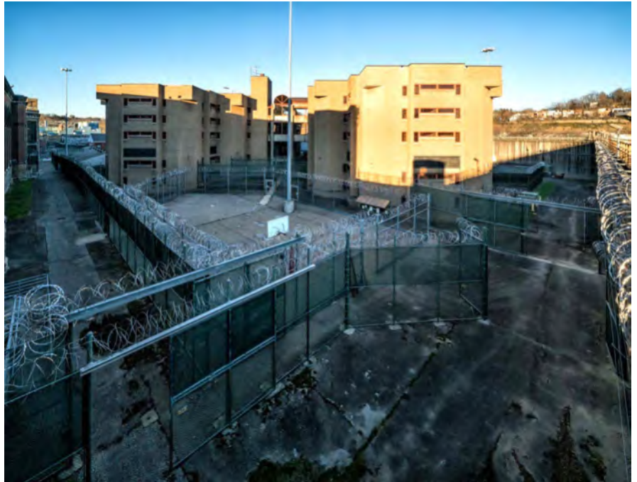
Photo 28. Housing Unit A/Building 5 (right) and Housing Unit B/Building 6 (left), looking northeast from Tower 7, showing recreation yards in the foreground.
