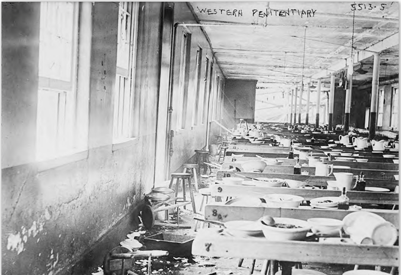
Figure 91. Photograph of the Dining Hall damage (Library of Congress).
