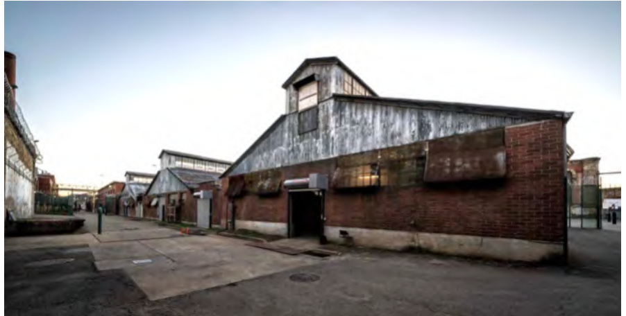
Photo 47. Correctional Industries Shop Building, looking southwest, showing (from right to left) the Welding Shop (13), the Metal Shop (12) and the Tag Shop (11).
