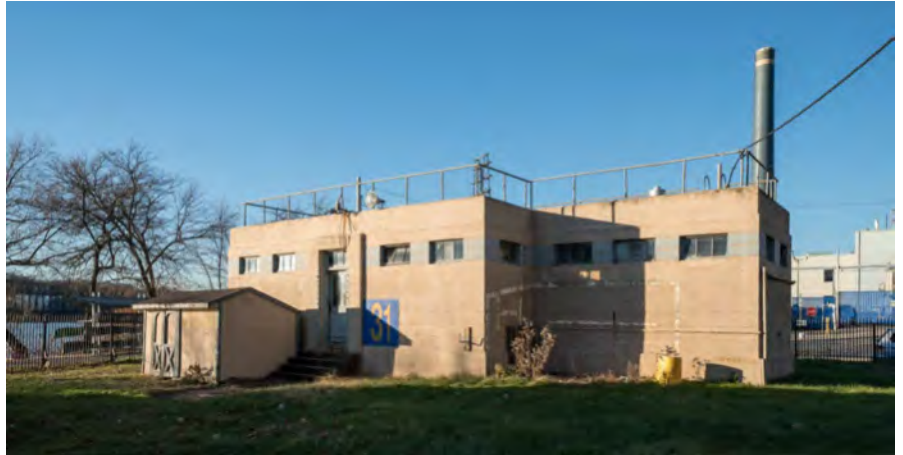
Photo 82. Sewage Pump House, south facade, looking northwest.
