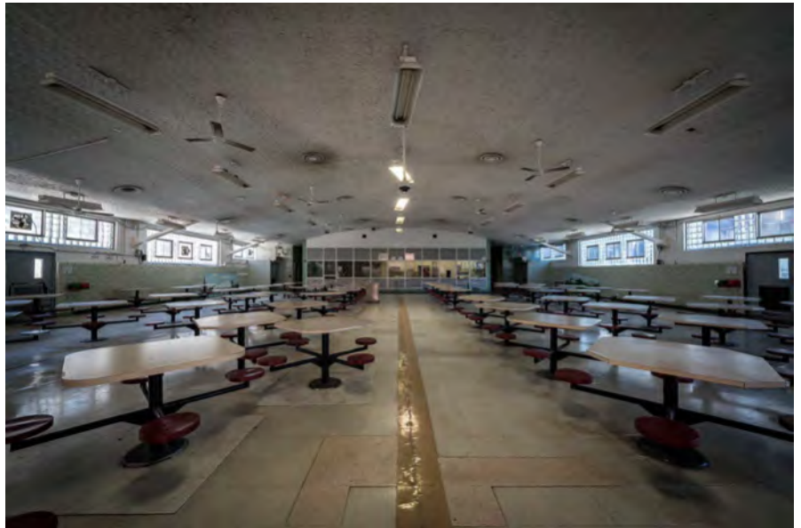
Photo 55. Dining Hall interior, looking south, showing the dining area. Above, the ceiling can be seen following the curved roof trusses (except at the perimeter where the ends of the roof trusses protrude).
