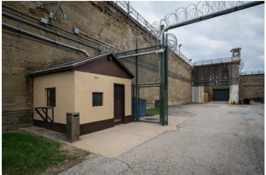
Photo 74. Scale House exterior, looking southeast.
