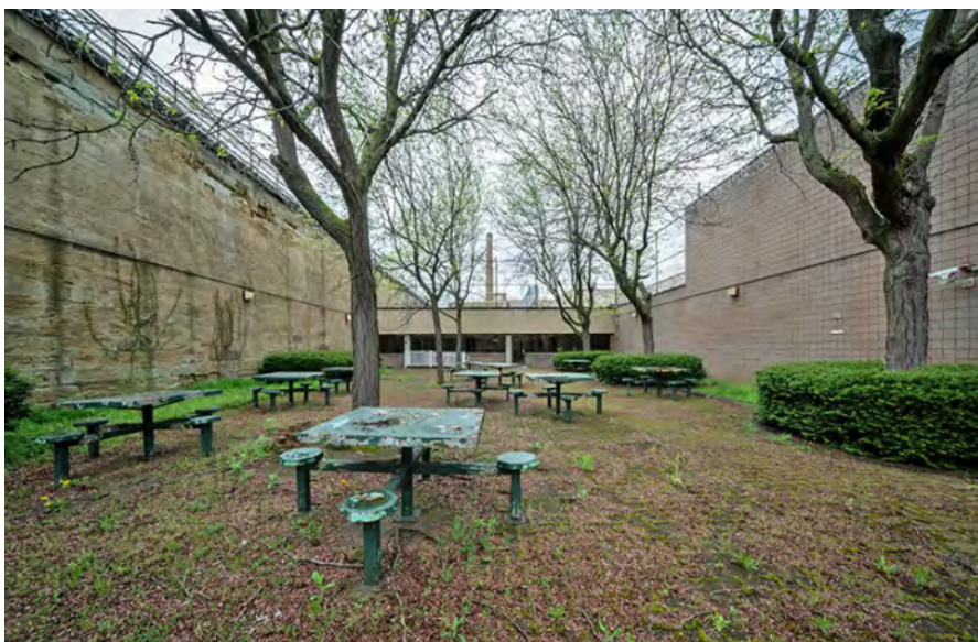
Photo 37. Administration and Visitors Complex, Visitors Courtyard, looking north, showing the original west wall of the penitentiary (left) and the visitor day room in the background.
