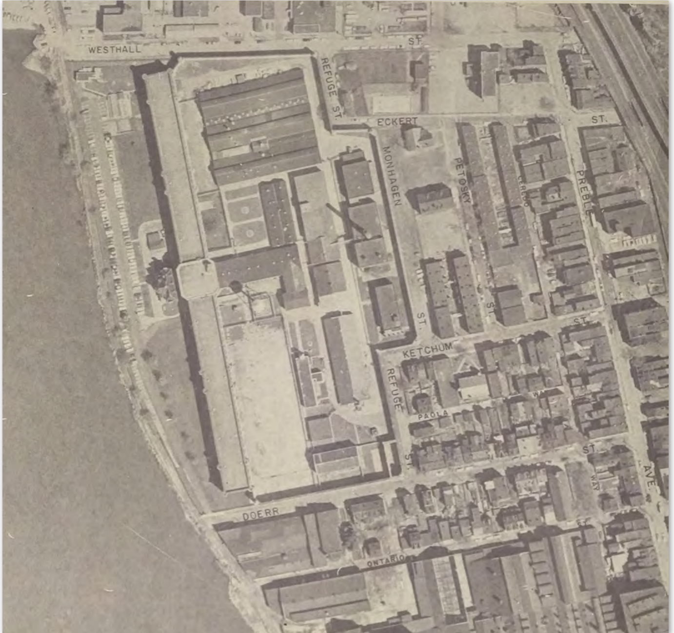
Figure 102. 1962 aerial showing the removal of the main penitentiary building's Victorian roof. The photo also shows that the ca. 1870 house portion of the Female Ward was demolished. The Sewage Pump House, located in the northwest corner outside of the Secure Perimeter, is also shown (Aerial Map Service Company, Pittsburgh, PA; obtained through SCI-Pittsburgh Facilities Archive).
