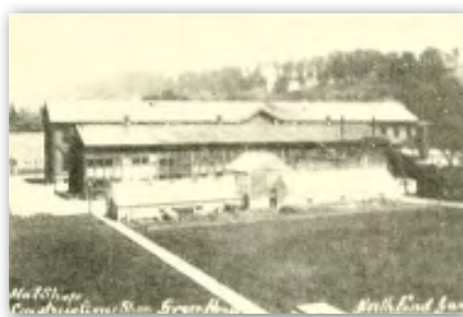
Figure 114. Photograph of the North Yard in 1897, showing several of the labor shops. From front to back, the Greenhouse, Machine Shop (also called the Construction Shop) and the Mat Factory (Mylin, State Prisons, Hospitals, Soldiers' Homes).
