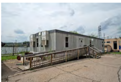
Photo 95. Modular Building southwest of Sewage Pump House, looking northwest.
