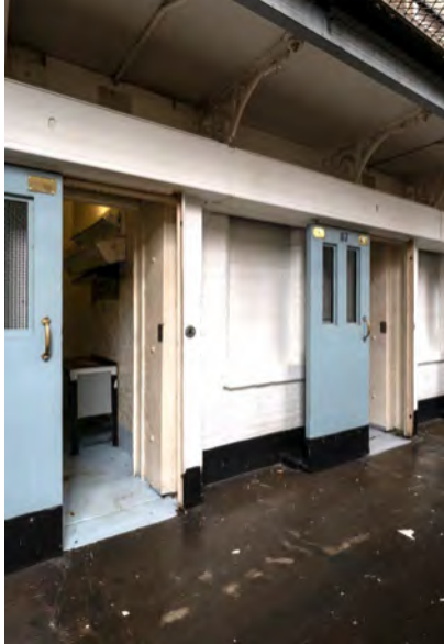
Photo 20. Main Penitentiary Building interior, Housing Unit C, looking east, showing a typical original window opening into a cell (center) that was filled with concrete block ca. 1983.
