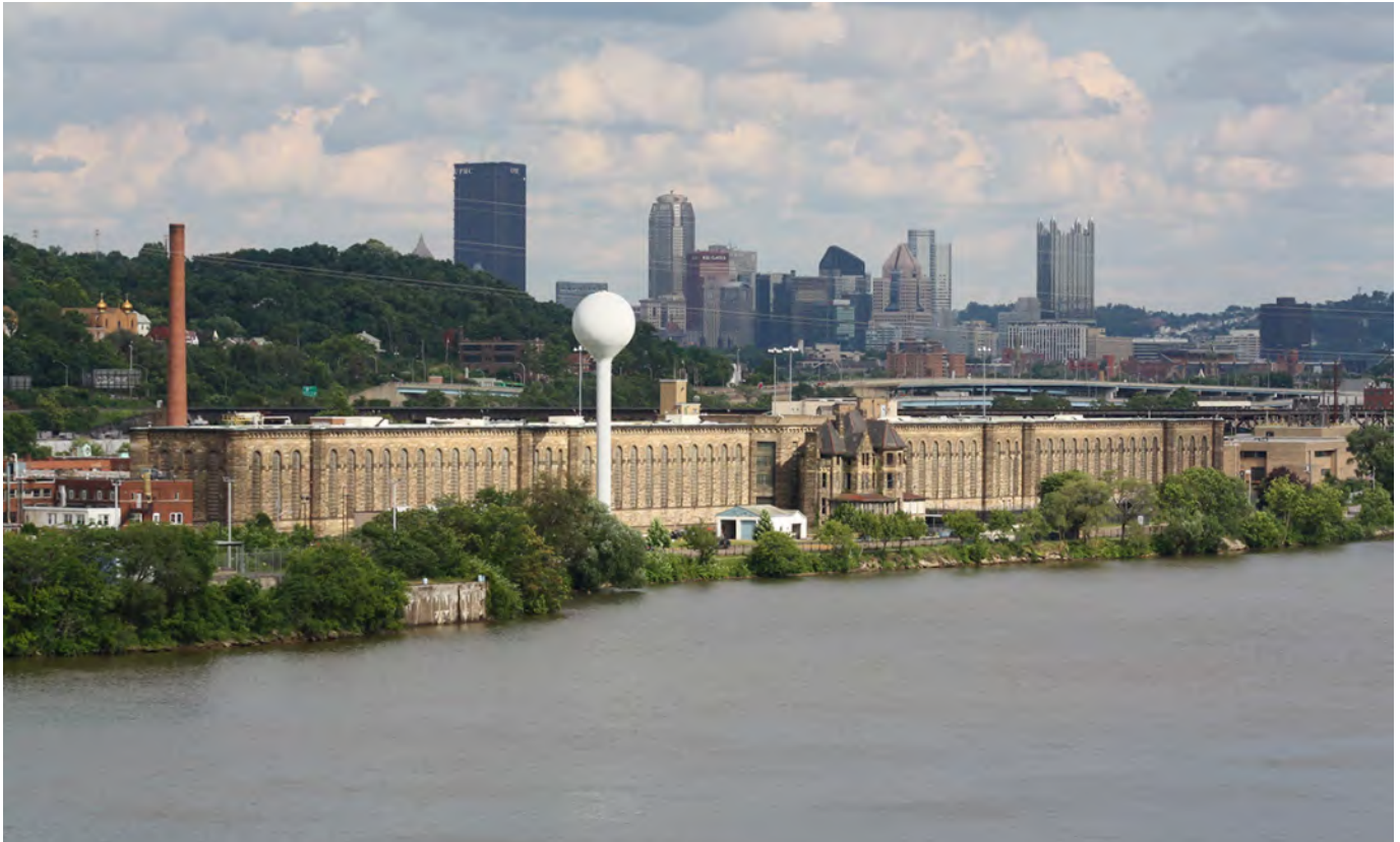
Photo 1. Western State Penitentiary, front facade, looking southeast, showing the close proximity to the Ohio River in the foreground and Downtown Pittsburgh in the background (Charles Rosenblum).
