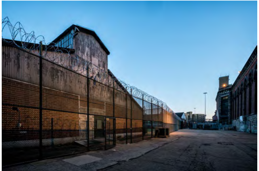
Photo 48. Correctional Industries Shop Building, looking south, showing the Tag Shop (11) at left.
