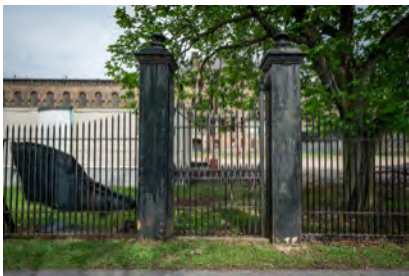
Photo 92. Cast and wrought iron gate, west side of Historic Front Yard, looking east, with the Warden's Residence in the background.
