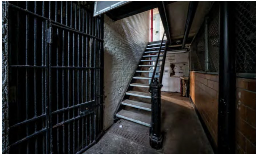
Photo 24. Main Penitentiary Building interior, Housing Unit D, first floor, looking northeast showing a typical stairwell.
