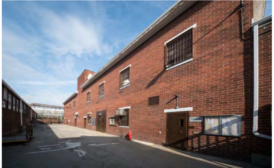
Photo 63. Library, Chapel and Education Building, west facade, looking northeast.
