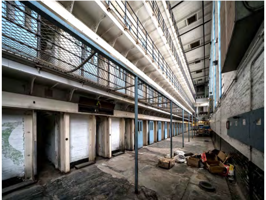
Photo 17. Main Penitentiary Building interior, Housing Unit E, North Wing, looking south, showing the five tiers of cells (left) set back from the exterior wall. The wire mesh ceiling (upper left) was installed to protect staff from thrown objects.
