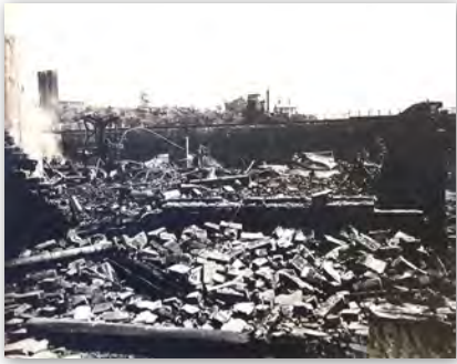
Figure 31. Remains of the historic East Wing, looking east, after rioting inmates burned down most of the buildings in the north half of the Secure Perimeter in 1921. The current building was rebuilt on this site (PA State Archives).
