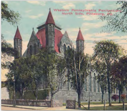
Figure 122. 1905 detail of roofline of Western Penitentiary showing High Victorian Gothic elements. The red color of the roof slates is speculation by the artist who colored the original black-and-white image for the post card.
