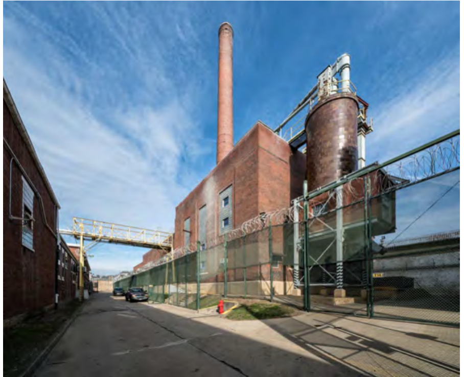
Photo 78. Exterior of Power House (right) and Boiler Plant (connected at left), looking northeast, showing the elevated site and foundation that aimed to keep equipment above flood waters.
