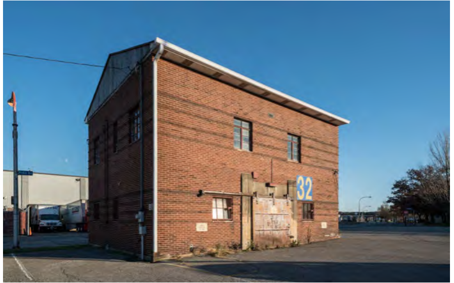
Photo 85. Maintenance Storage Building, exterior, looking southwest.
