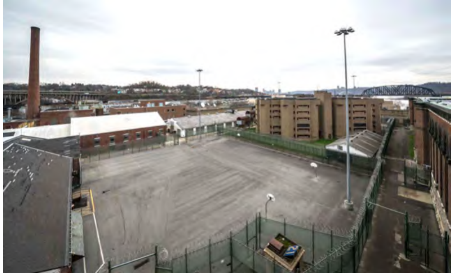
Photo 5. South end of the Secure Perimeter, looking southeast from the roof of the Rotunda, showing the Main Yard (center).
