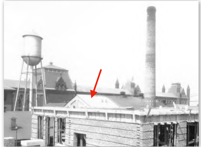
Figure 47. Detail from a ca. photo, looking northwest, showing construction of the old hospital in the foreground and the new south addition to the Gymnasium. Note that the 127-foot chimney of the old electric plant has not yet been removed (University of Pittsburgh Archives).
