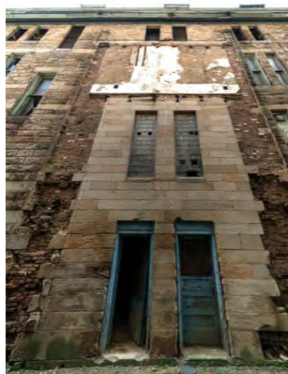
Photo 8. Warden's Residence, rear facade, looking west, showing where the porte cochere and bridge once existed.
