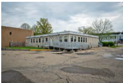
Photo 99. Staff Lockers / Wellness Center (42), looking northeast.
