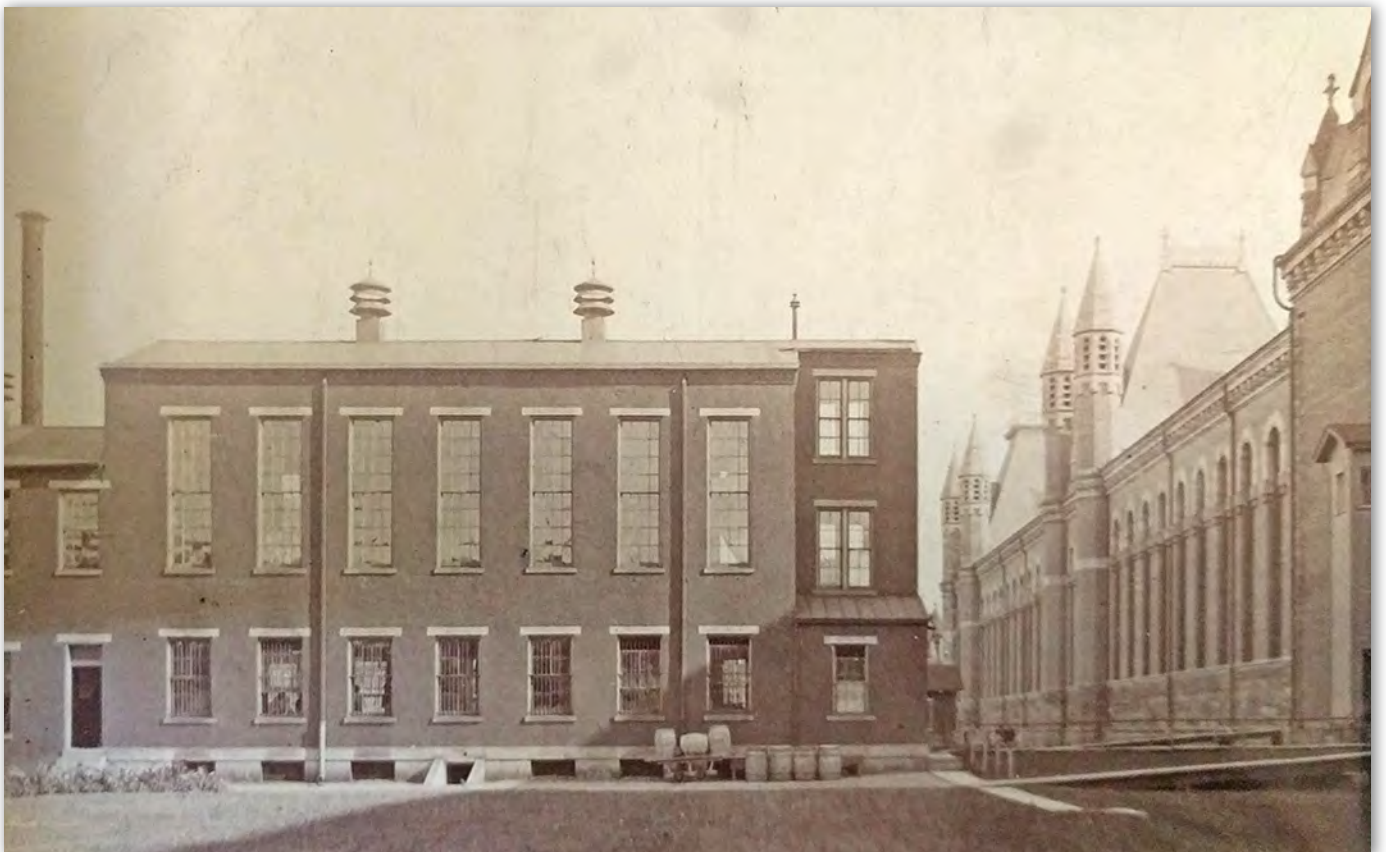
Figure 76. Ca. 1890 photo showing the East Wing of the former House of Refuge that Butz incorporated into his design. At the time of this photo, the main block of the House of Refuge has been demolished, leaving a gap between the East Wing and Main Penitentiary Building. By 1893, the stair tower (right end of East Wing) was removed and a connector was built joining the East Wing and the Rotunda (PA State Archives).
