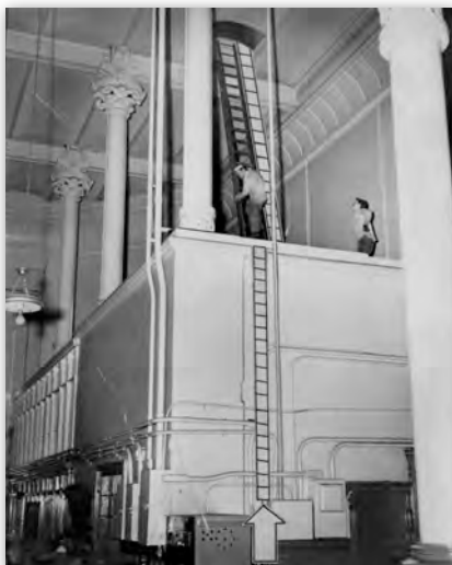
Figure 26, showing the escape route through the upper floor of the Rotunda taken by inmate Andrew Kaczynski in May 1951 (he was recaptured a month later). Note the clear ceiling height of over 35 feet—this was two years before the floors were inserted for the diagnostic and classification center (Pittsburgh Post-Gazette).
