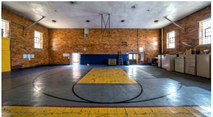
Photo 59. Gymnasium interior, looking south, showing the playing surface and primary entrance doors.
