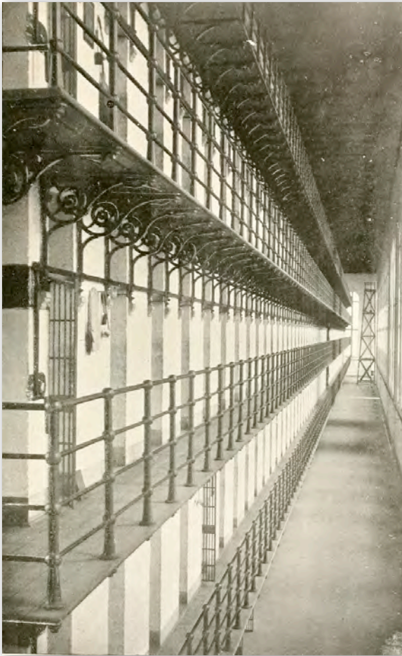
Figure 24. Cells in the South Wing in 1897. Note the original iron-barred door (left), the ladder/scaffold that was employed to open and close the original windows (right), and the uninterrupted length of the cell block (PA State Archives).
