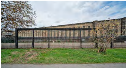
Photo 93. Large, sliding cast and wrought iron gates, west side of Historic Front Yard, looking east.
