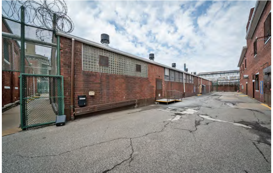
Photo 42. Services Building, east facade, looking northwest.
