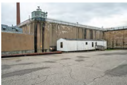
Photo 102. Corrections Emergency Response Trailer, looking southwest.
