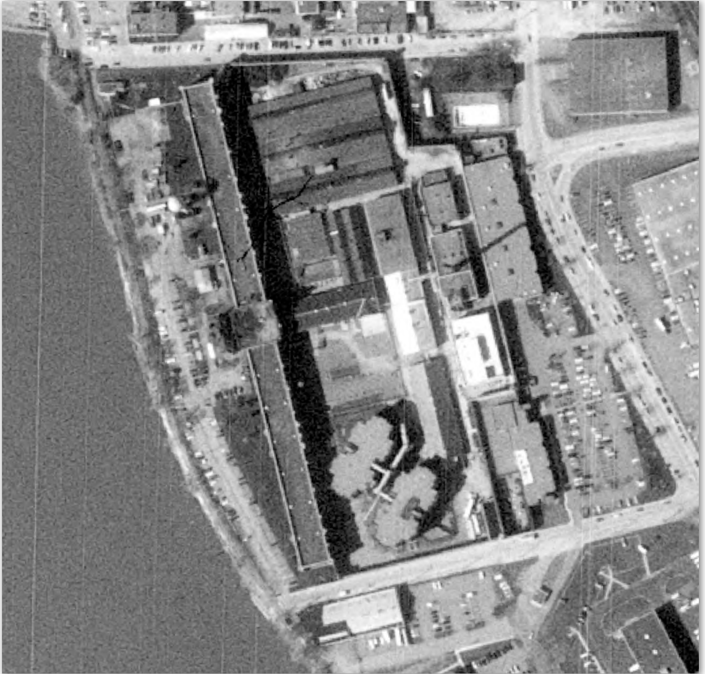
Figure 107. 1993 aerial photograph showing major changes to the site under the 1984 master plan by architect Tasso Katselas. Under this plan, two new cell blocks were constructed in the southern end, along with the Administration and Visitors Complex and the Institution Warehouse, which were built along the eastern side of the Secure Perimeter. The main penitentiary entrance shifted to the eastern side of the site.
