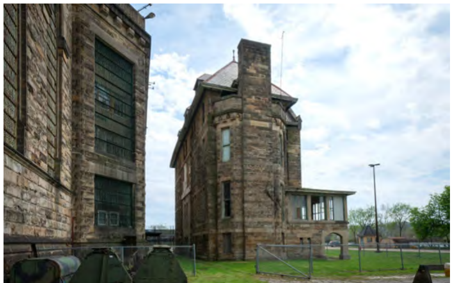
Photo 9. Warden's Residence, north facade, looking south, showing the narrow gap between the house and the Main Penitentiary Building. Also visible is one of the three-story, octagonal bay windows with integral end chimney.
