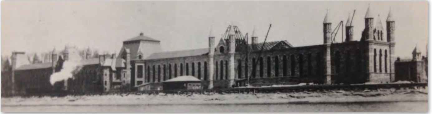
Figure 75. 1893 photo showing construction of the roof over the South Wing. Inmates were already being housed in the wing at this time (Carnegie Library of Pittsburgh).
