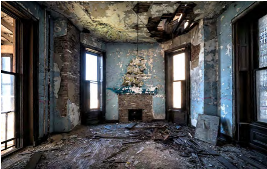
Photo 11. Warden's Residence interior, dining room, looking north, showing the brick bearing wall construction (left), missing mantel with mural above (center) and remaining window trim throughout (including interior shutters).
