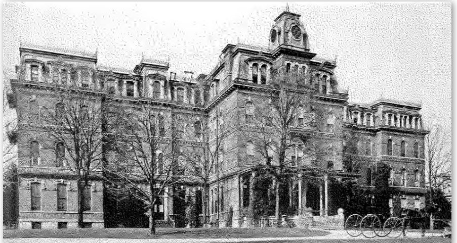
Figure 17 The Administration Building at the Pennsylvania Reform School at Morganza (1873-1927).
