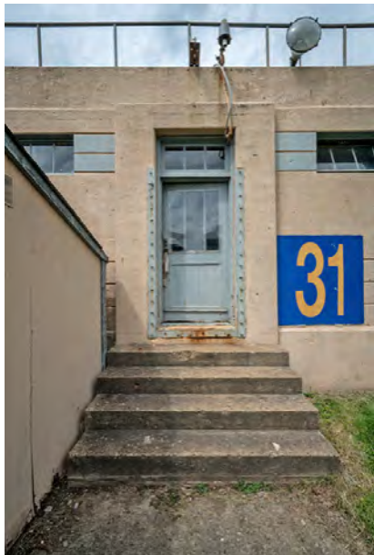
Photo 83. Sewage Pump House, detail of front entry, looking north.
