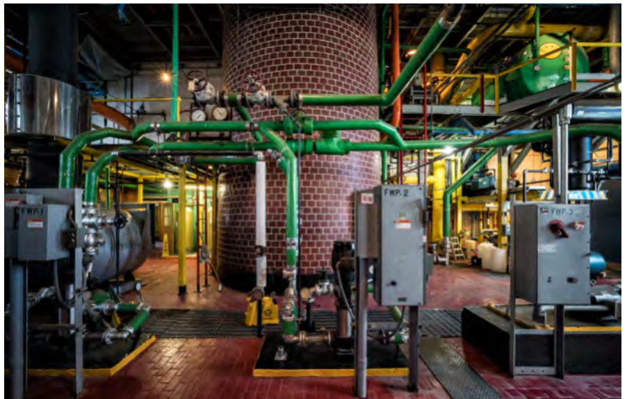
Photo 79. Boiler Plant interior, looking south, showing the base of the smokestack.
