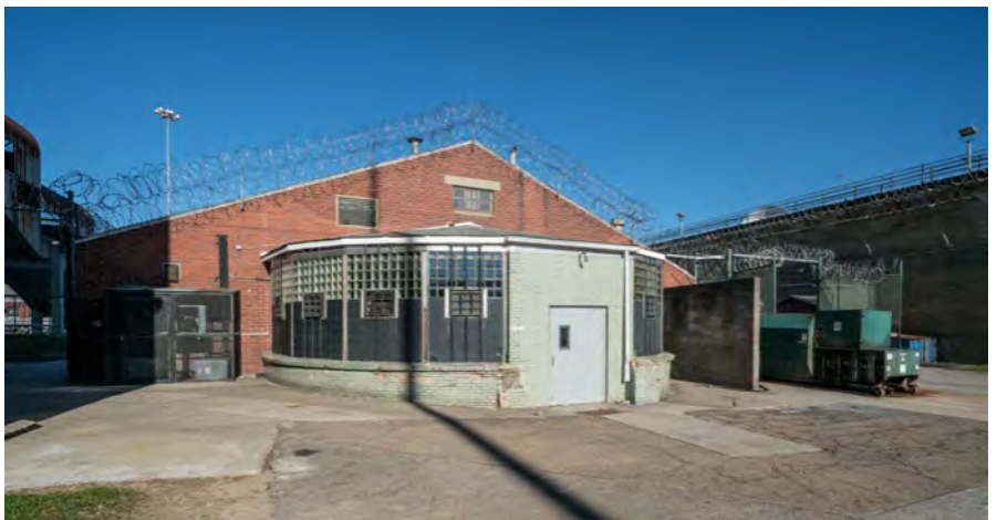
Photo 54. Dining Hall, south facade, looking northeast, showing the red brick south wall of the 1957 addition and the half-round dish washing room in mint green glazed brick and glass block.
