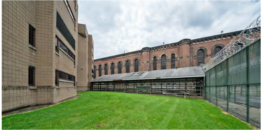
Photo 67. Exercise Pavilion (center), looking west.
