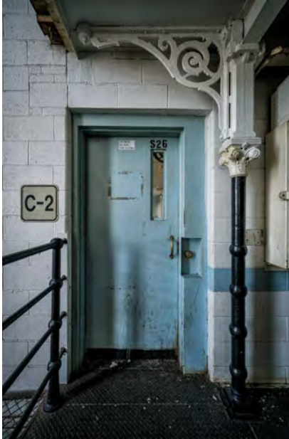
Photo 104. Examples of structural and ornamental cast iron found throughout the Main Penitentiary building. The Female Ward had similar details.
