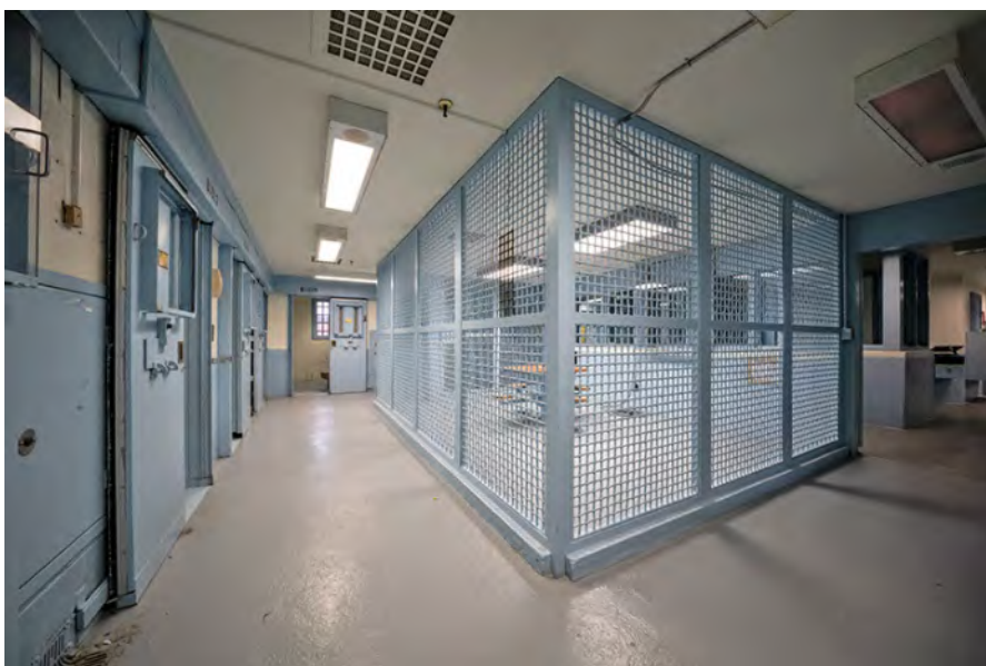
Photo 33. Housing Unit A/Building 5 interior, second floor, showing a smaller cluster of cells and a higher level of security (e.g., steel mesh-enclosed day room) than found in Housing Unit B.
