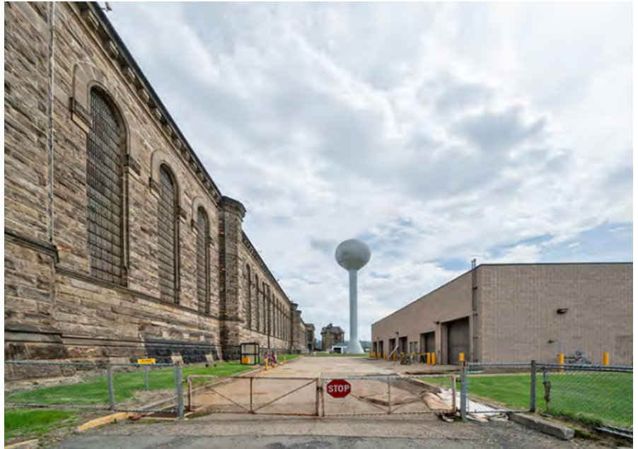
Photo 86. Vehicle Maintenance Building exterior (right), looking south.
