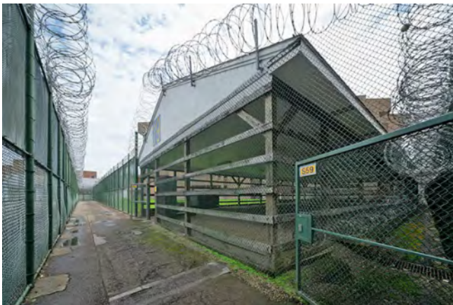
Photo 68. Exercise Pavilion, looking southeast.
