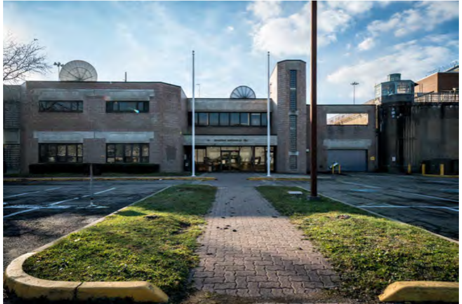
Photo 34. Administrative and Visitors Complex, east facade, looking west, showing the vehicle access door (at right) where prisoners would enter the facility for processing.
