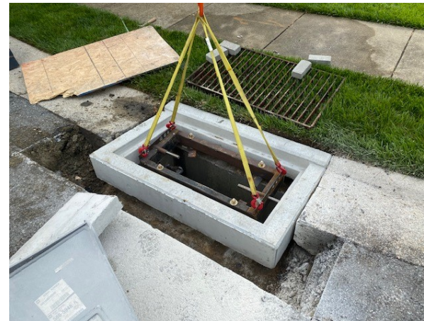
2023 State Winner: Inlet Replacement Tools London Grove Township, Chester County
