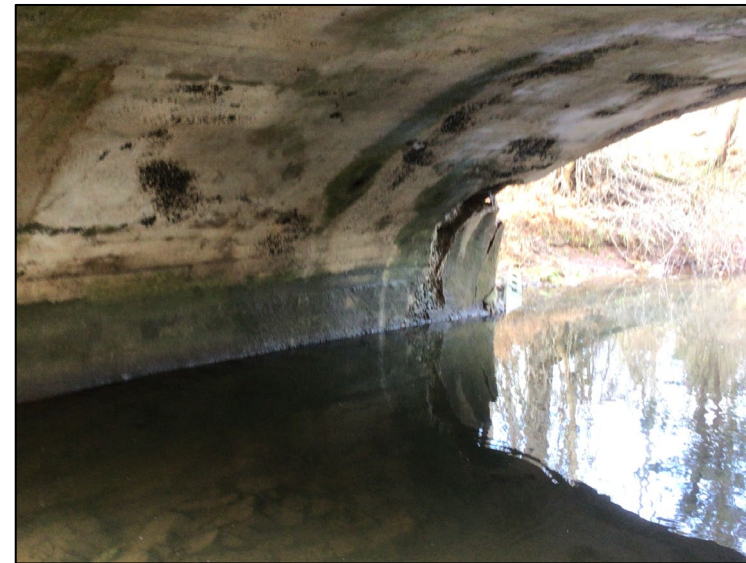
Underside of arch looking southwest
