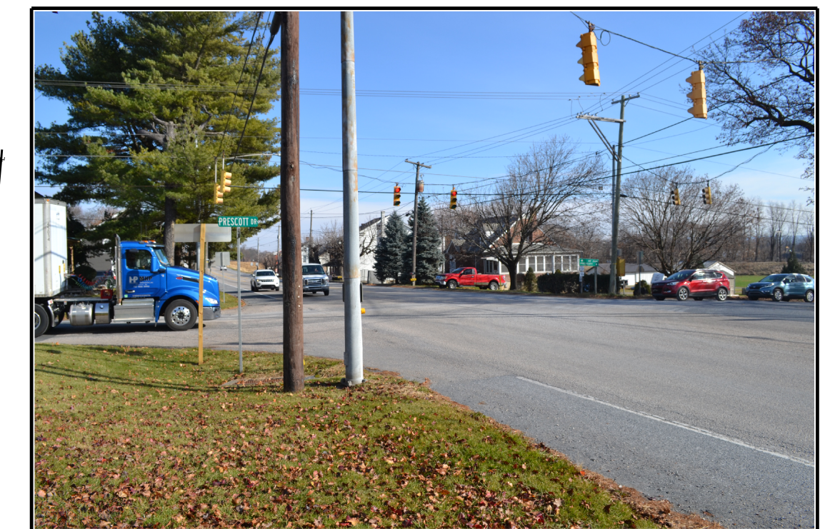
EXISTING INTERSECTION (LOOKING EAST)
