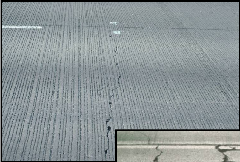
CRC Transverse Cracking
