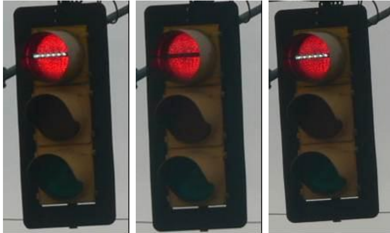
Exhibit 4-31 Traffic Signal White Strobe Lights
