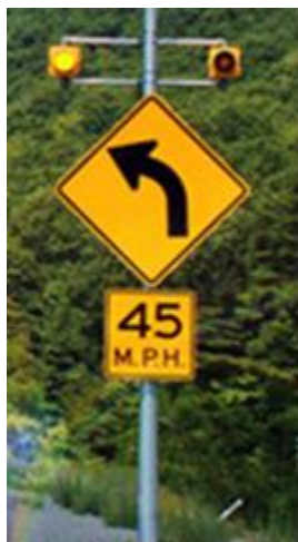
Exhibit 4-16 Curve Ahead Warning System
