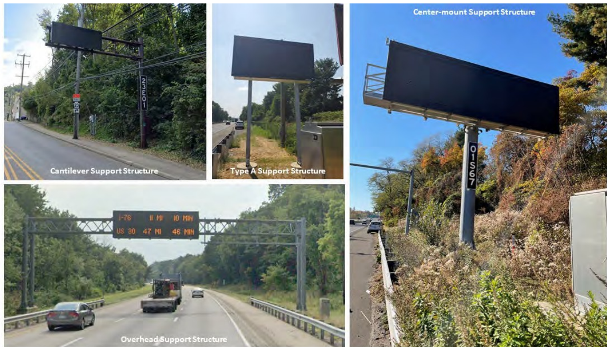
FIGURE 15: CMS SUPPORT STRUCTURES
