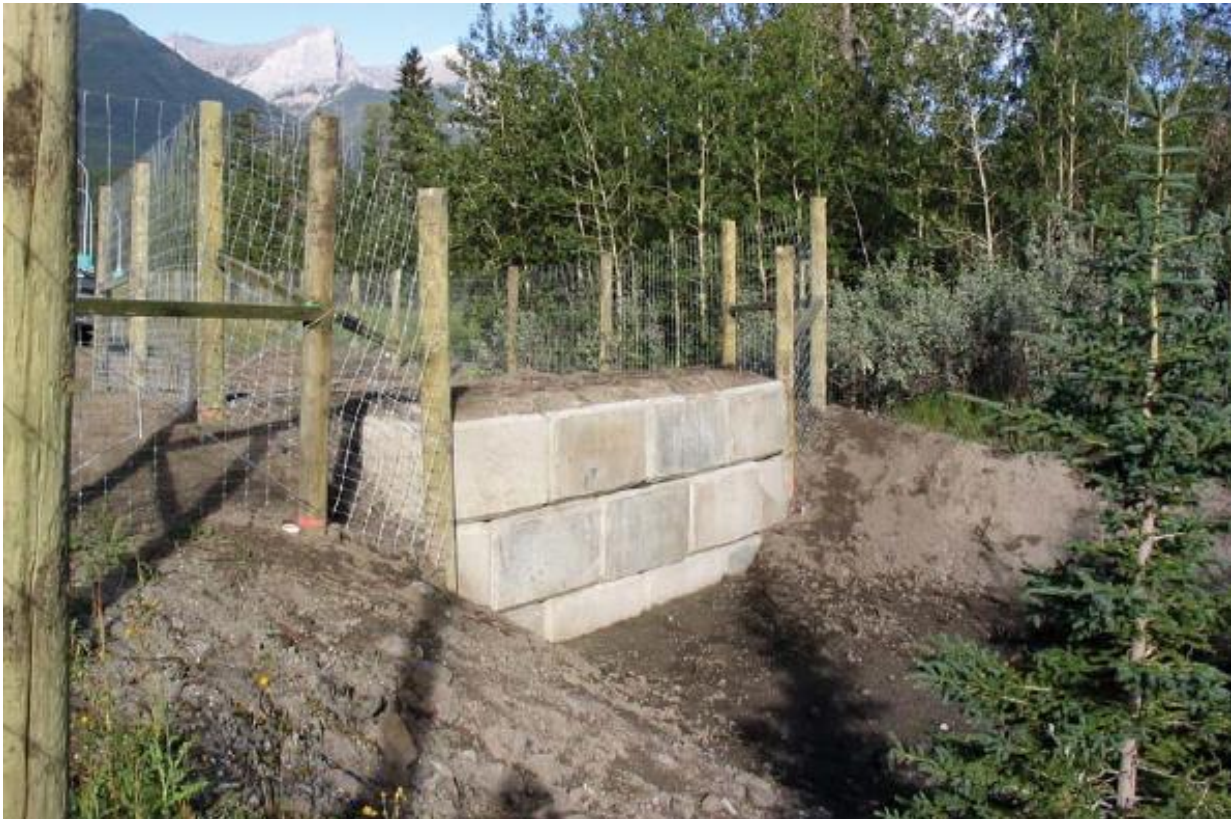
Example of "Jump-out" Structure
