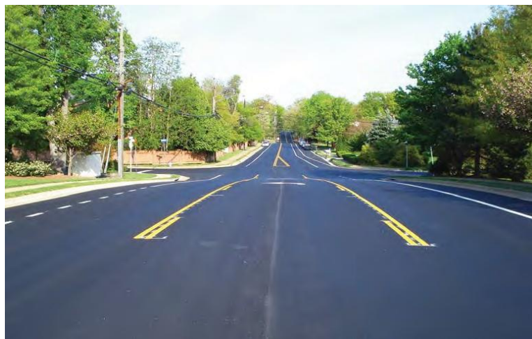
Exhibit 8.6.2 Transition from Three-Lane to Two-Lane
