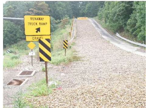
Guide rail is shown above, but is not required on escape ramps.
