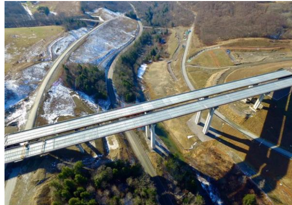
Viaduct Underpass (U.S. 219 PennDOT District 9)
