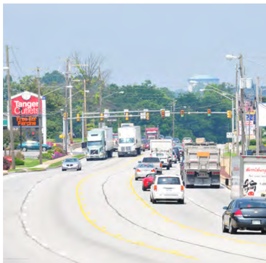
Typical roadway section with center turn lane
