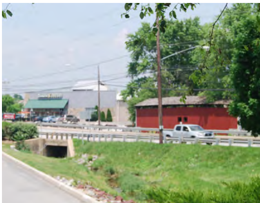
Drainage area at Rockvale Outlets
