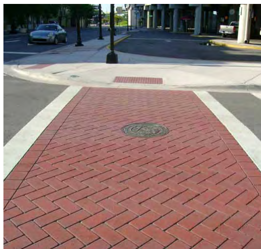
“TrafficPatterns XD” style thermoplastic pavement marking applied and stamped into the asphalt surface
