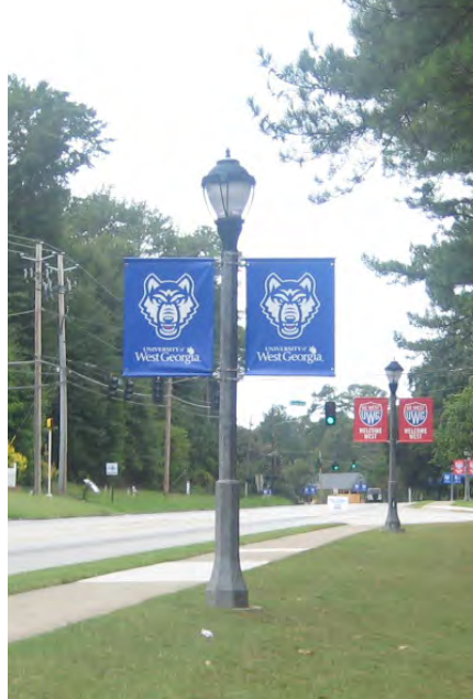
Pedestrian lighting with banner sign
