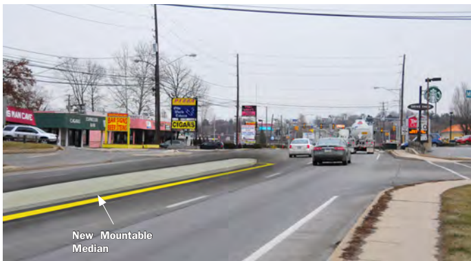
Phase 1: Installation of median to prevent left turns from Millstream Road
