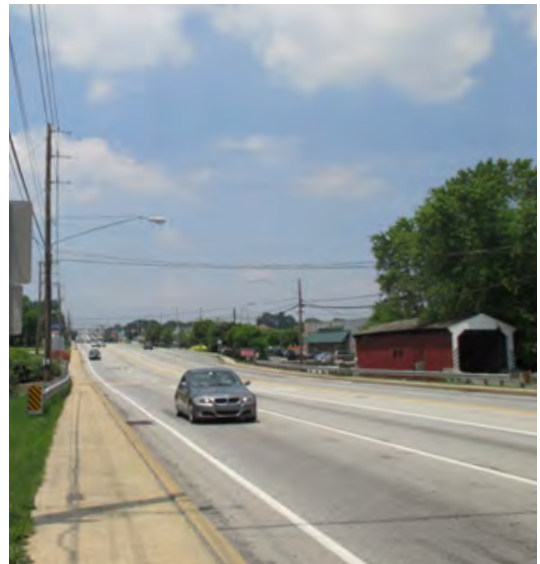
Bridge structure at Rockvale Outlet
