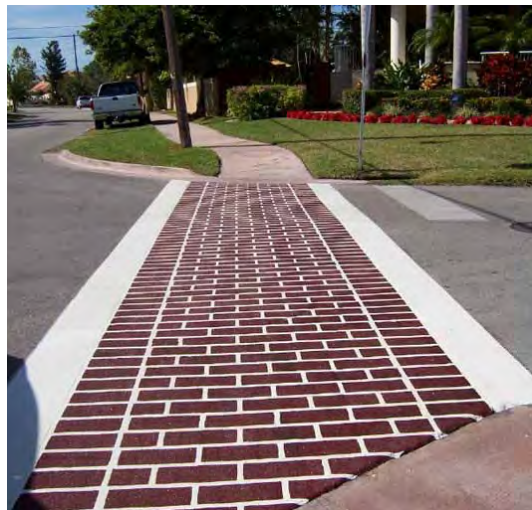
“TrafficPatterns” style thermoplastic pavement marking from TrafficScapes applied to flat asphalt
