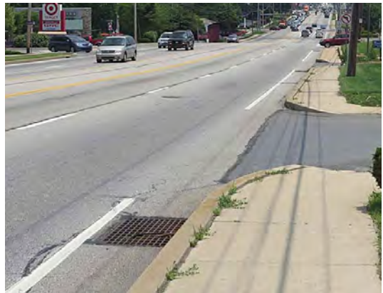
Stormwater grate at Travelodge entrance
