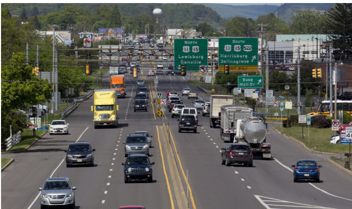
A congested section of Route 15 looking north to Shamokin Dam. Access management programs and ordinances can reduce traffic conflicts and reduce congestion. Photo credit: Mark Pynes.
