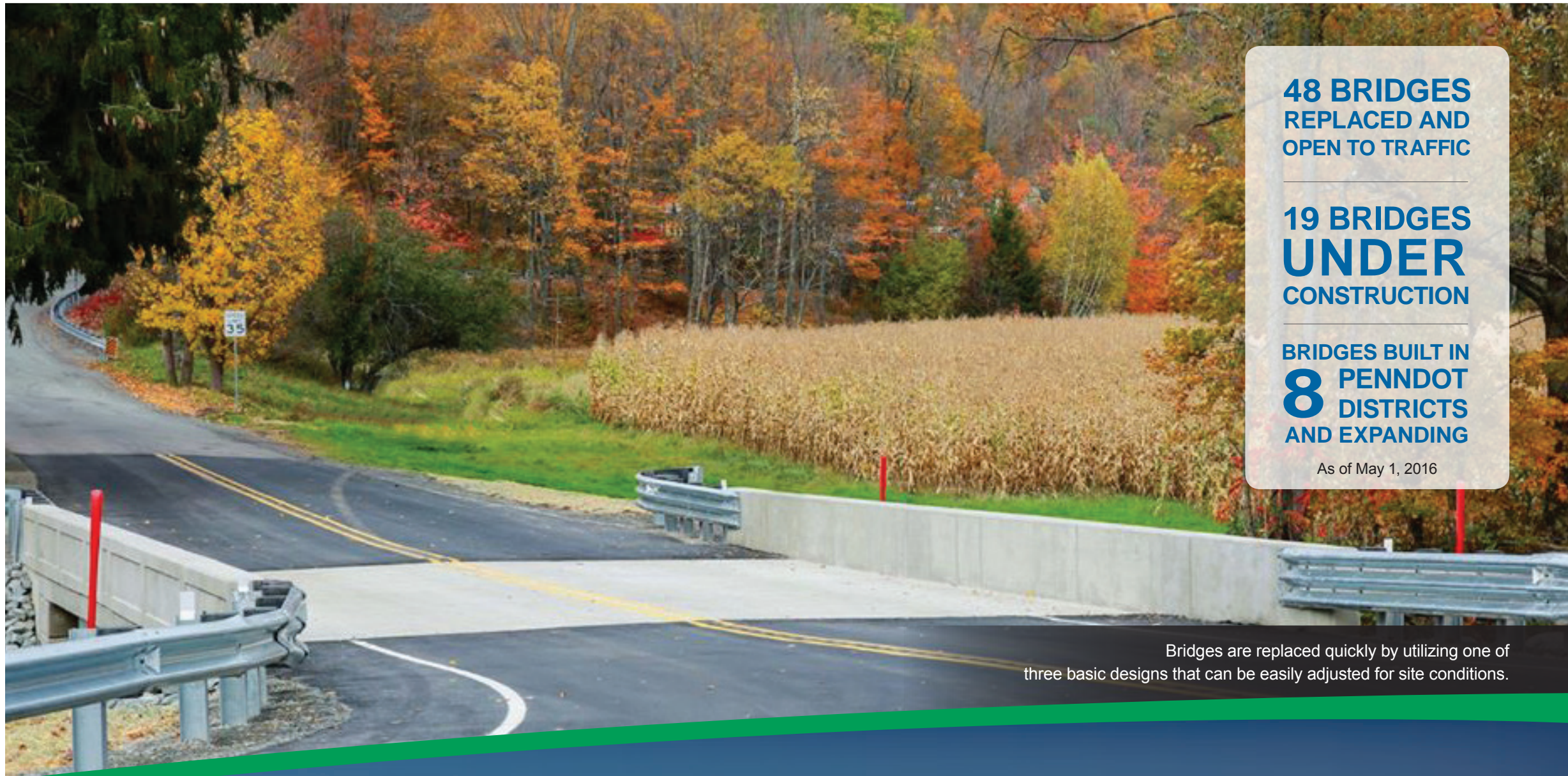
PennDOT's Rapid Bridge Replacement Project successfully completed more than 40 bridges in its first year.
