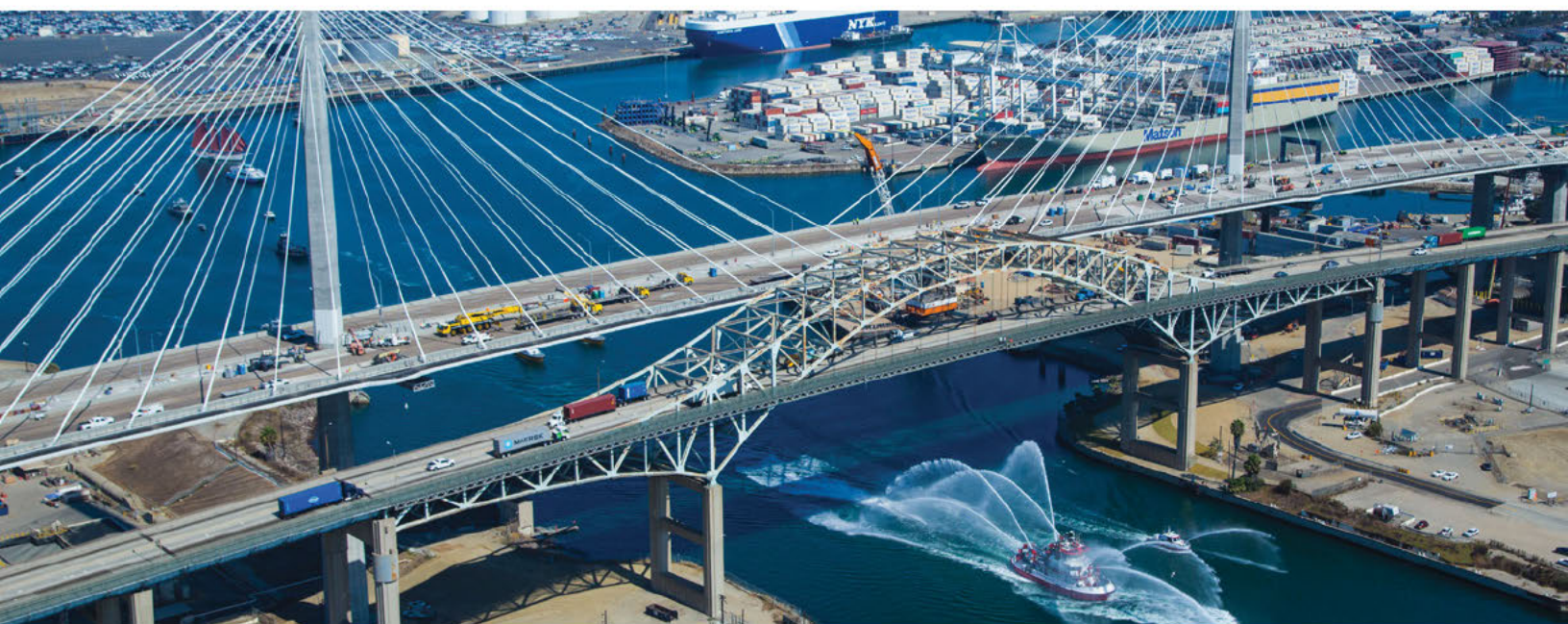
Gerald Desmond Bridge, California FCC
