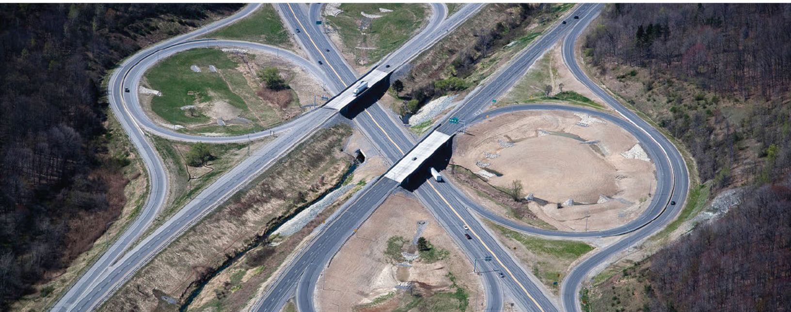
I-79 Meadville Interchange Reconstruction, Pennsylvania Fay
