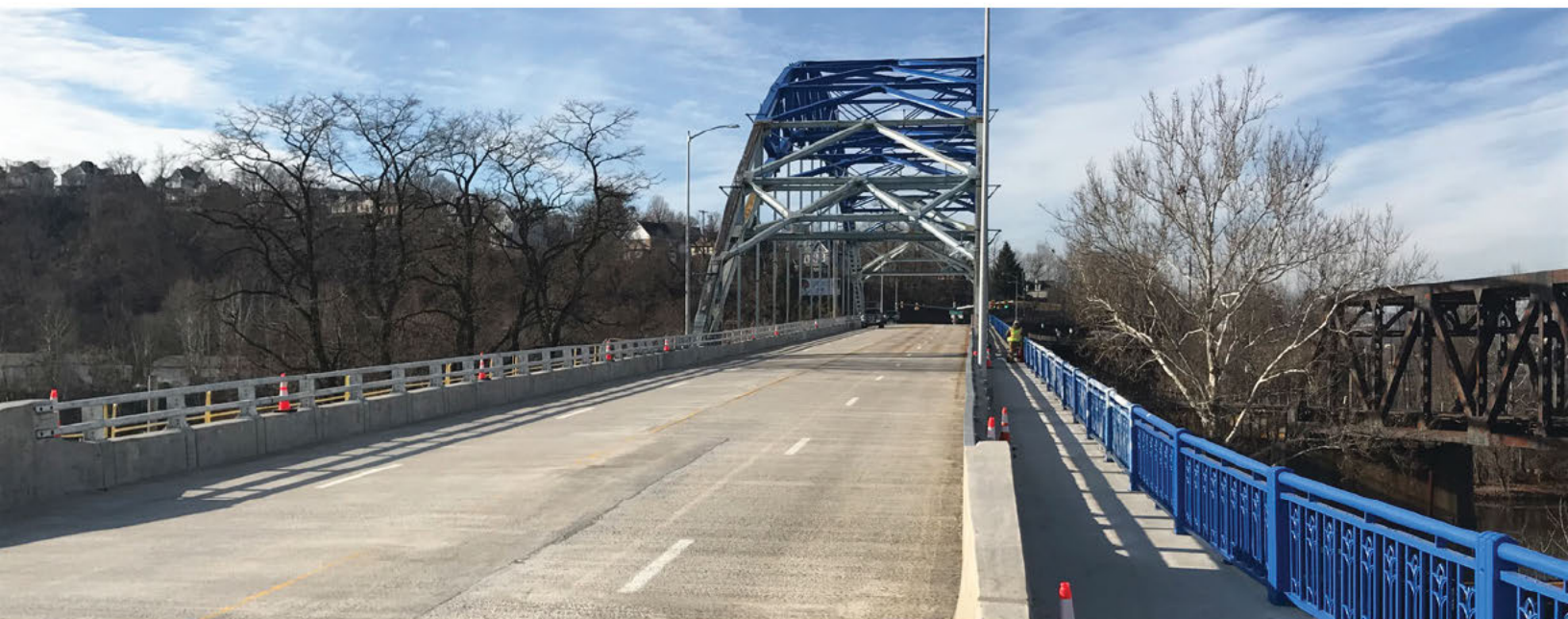
Jerome Street Bridge Rehabilitation, Pennsylvania Fay
