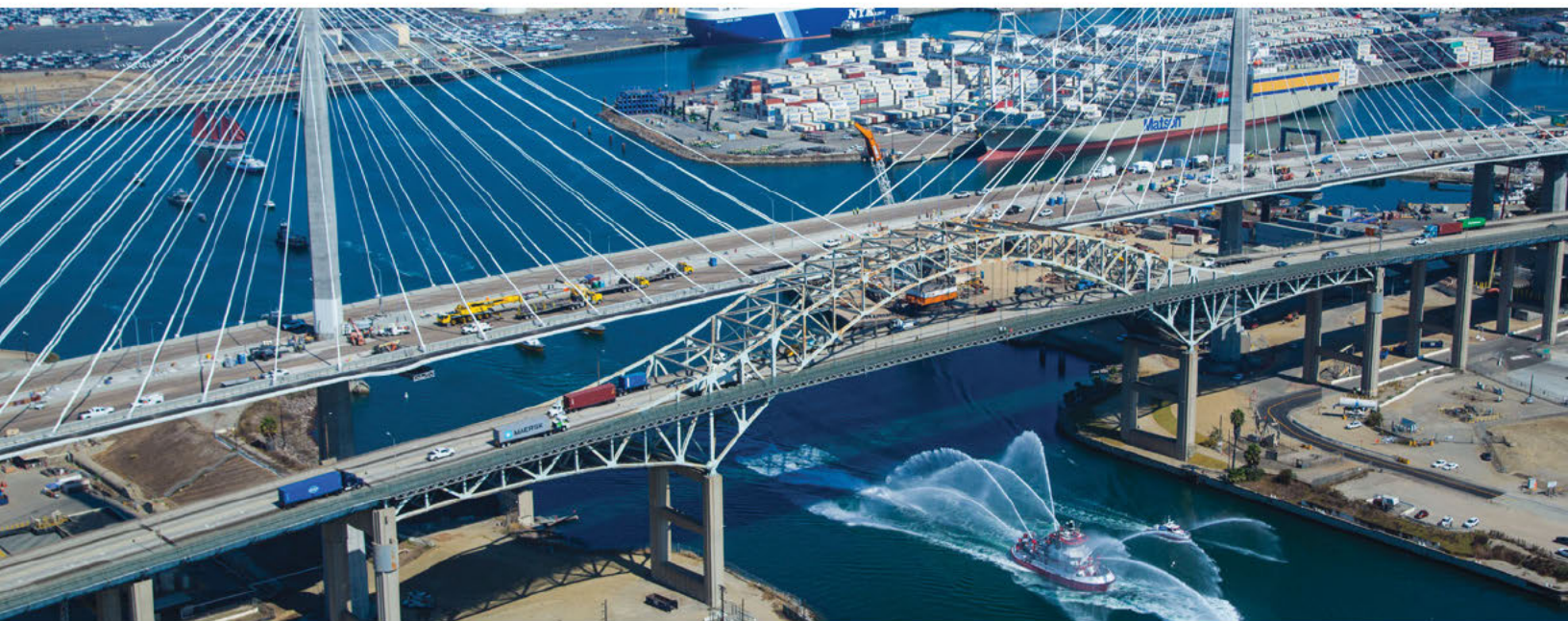
Gerald Desmond Bridge, California FCC
